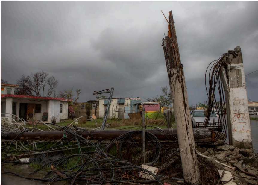
Damage to utility poles in Puerto Rico
