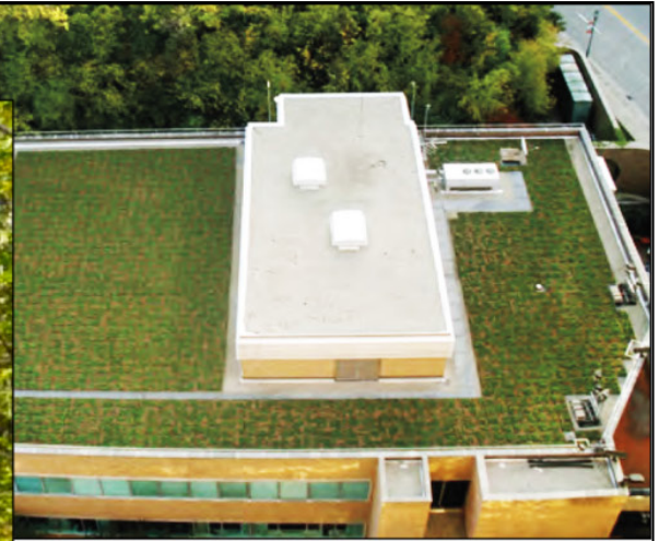
Green roof – a roof either partially or completely planted with vegetation growing in soil (or a growing medium) to hold rainwater.
