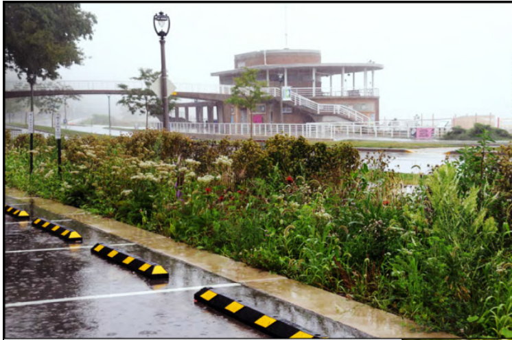
Bio-swale – a depressed catchment area planted with vegetation that captures and infiltrates runoff.
