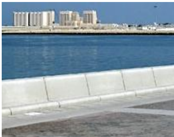
Figure 15. Example of parapet wall
