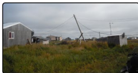
Thawing permafrost undermining electricity infrastructure in Newtok
